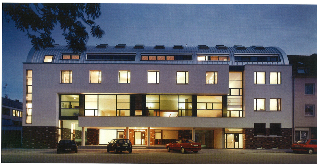
10.35 The new building to the north, adorned with a curved metal roof, protects the bunker units behind and extends the complex to meet the street
